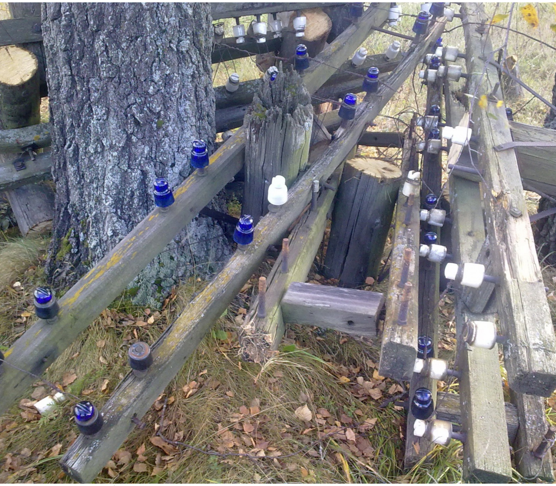
COBALT 565.1S ON RECENTLY ABANDONED TELEPHONE CIRCUITS. PHOTO FROM ALEXANDER BULBA AT USSRINSULATORS.COM
