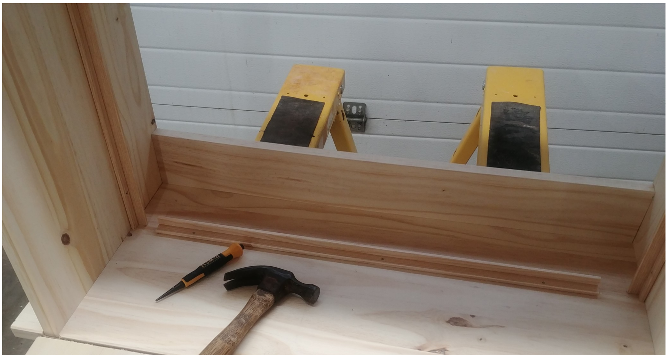
Figure 18: A small tack hammer and a nail punch should be used for driving in the wire nails that will hold the L-shaped moulding. This moulding will then hold the light panel in place, so the nails must be driven down flush without damaging the moulding.
