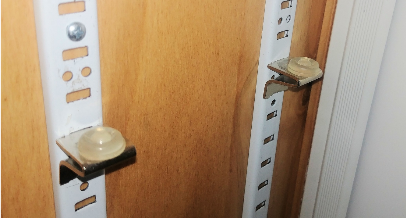
Figure 48: The rubber pads on the clips help the shelf seat firmly. Without them, any unevenness in the shelf standards will cause the shelf to rock back and forth, clanking every time.
