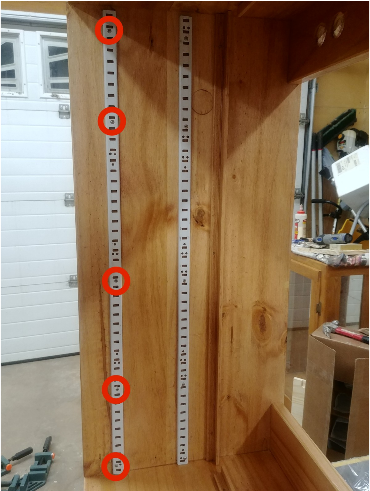
Figure 23: Put screws in the holes circled in all standards to avoid conflicts with common shelf heights.
