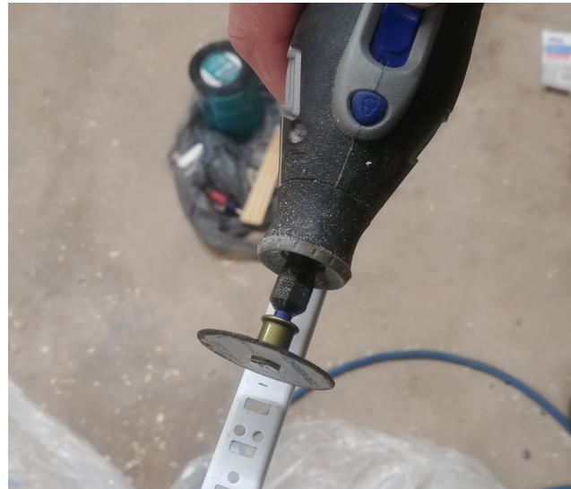
Figure 22: A Dremel carbon fiber cutoff wheel makes quick work of the standards, but be sure to wear safety glasses. This thing throws tons of tiny metal fragments.
