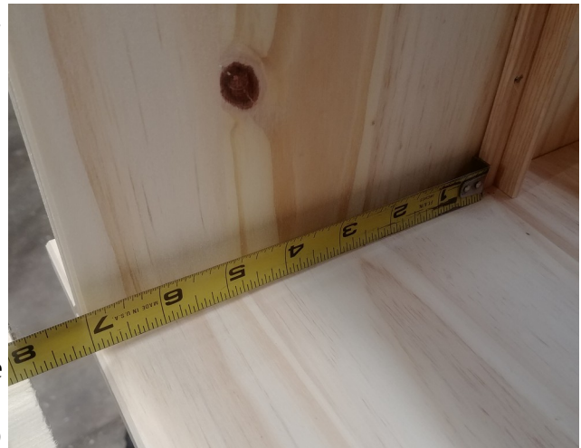
Figure 17: The front of the L-shaped corner moulding should be 7" from the cabinet front
