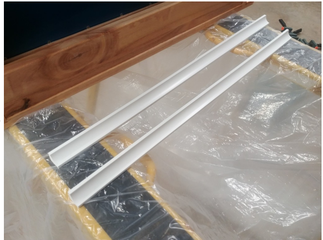
Figure 24: Two 23-3/5" PVC inside corner mouldings ready to be drilled
