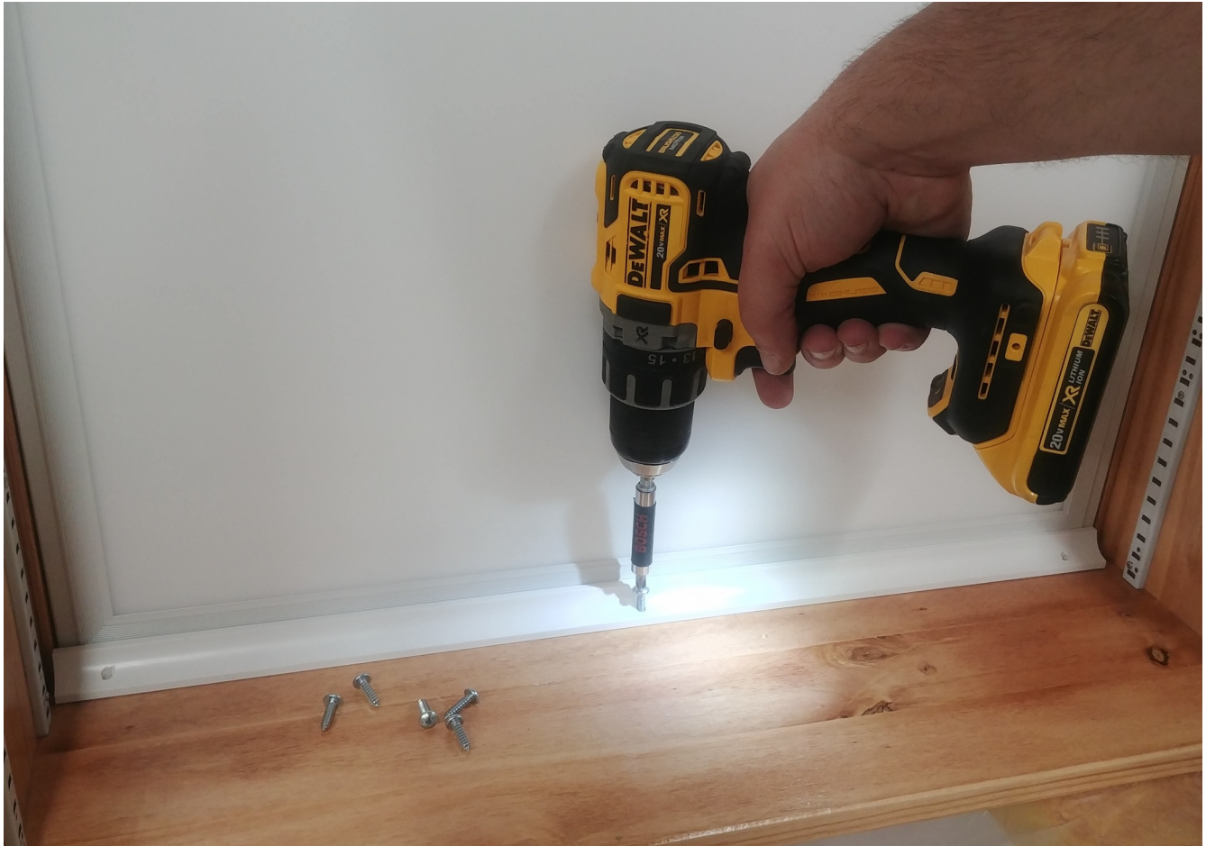
Figure 31: Install the two pieces of inside corner moulding tight up against the LED panel to hold it in place in the L-channel.
